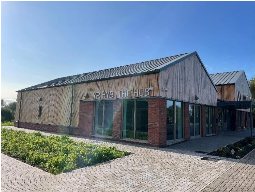
Image of Magor Community Hub partly funded via significant s106 agreement financial contributions from local developments allocated in the Local Development Plan (above); and the building as constructed in September 2023 (below)
